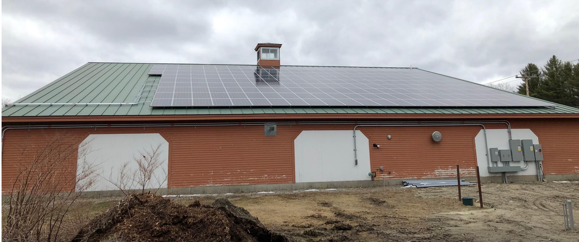
Photo: New London Municipal Solar Array - 210 panels on Highway Garage roof
